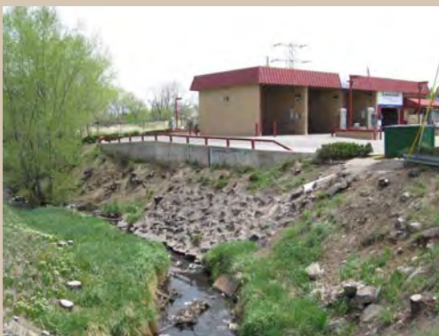
Drainages in the study area have been heavily modified by past development. While the US 6/Wadsworth project would destroy several small wetlands, proposed widening of gulches would improve conditions for new wetlands and natural riparian areas to establish.
