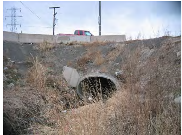
46 EXHIBIT 4-4: DRY GULCH CULVERT
